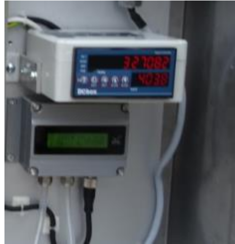
Fig. 2. Measurement panel (recorder and adder) of the flow meter used in new ASS-500 stations
